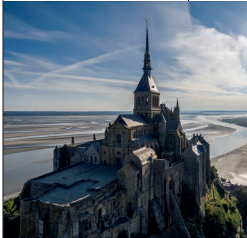
Mont-Saint-Michel Abbey, aerial view from the south-west
